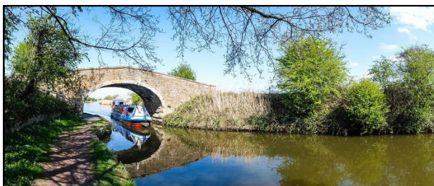
Bridge 24 at Halsall
